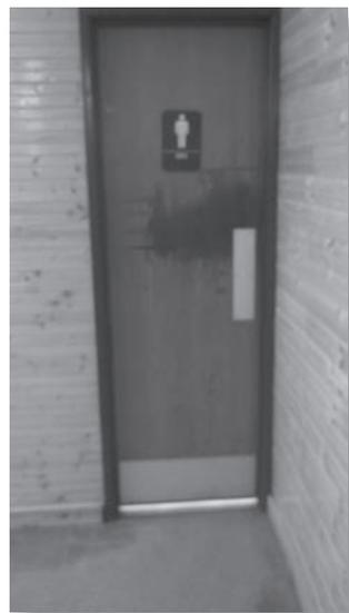
It is a bit hard to tell, but this restroom door is far too narrow. The ADA requires a 32 inch minimum clear opening space through the doorway. This one is barely wide enough to walk through, much less navigate in a wheelchair.
