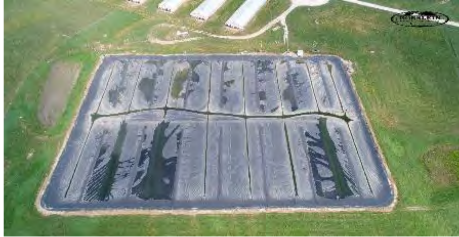
Covered waste lagoon at Valley View Farm, Missouri, 1.2 Hectare
