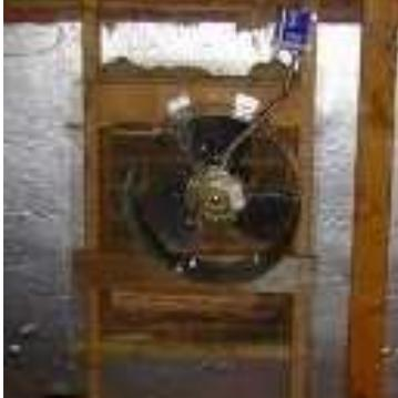
Simply install vertically using appropriate hardware. Mount against an existing gable vent. Put plywood, cardboard, or flat insulation material on the part of the gable vent that is not covered by a fan. (This will prevent backflow)
