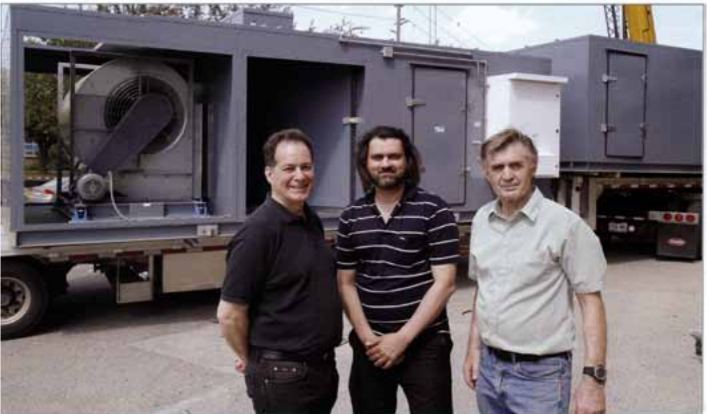
From left to right: Elliot Strashin (Strashin Developments), Imran Majeed (Advanced Building Solutions) and Dennis Campbell in front of BKM unit before being lifted to the 501 Alliance Ave. rooftop
