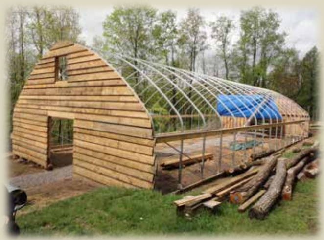
Installing the Hoops and Building the Wooden Ends
