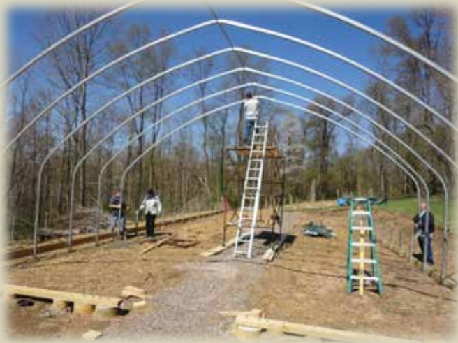
Installing the Hoops and Building the Wooden Ends
