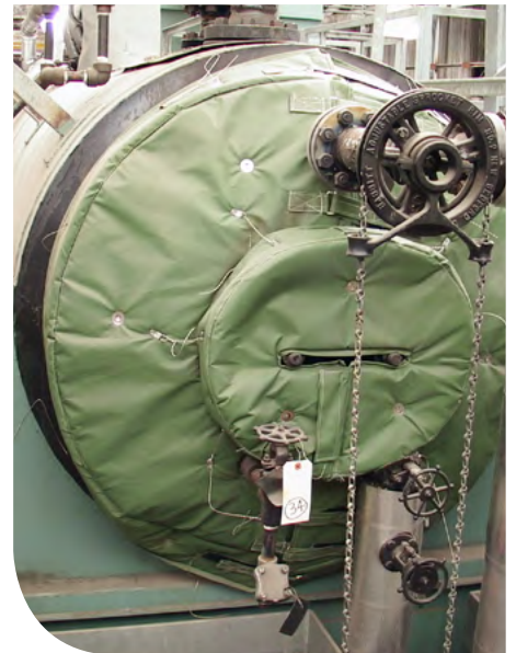
BOILER HEAD STEAM DRUM Design: Steam Drum Retrofitted with Blanket Fastener: Stainless Steel Wiretwists
