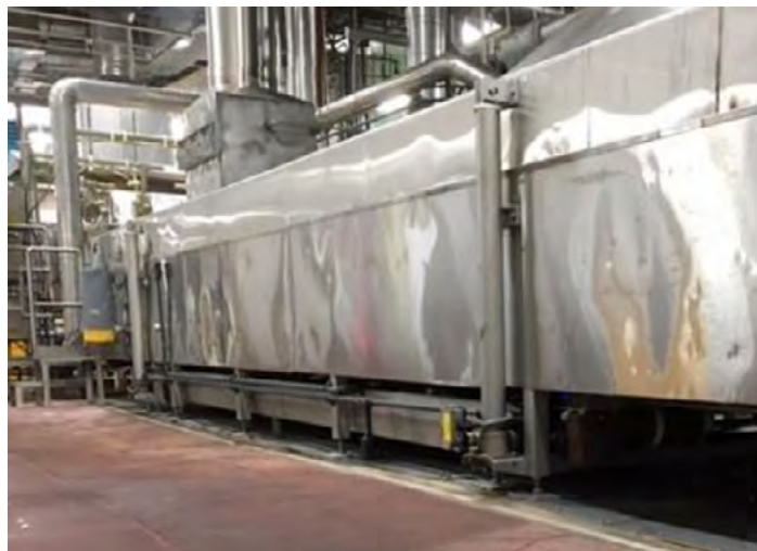
Hot Oil Fryer – Food Processing - Wash Down
