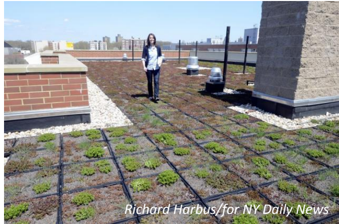
A WHEDCO program manager, Erin Burns walks on the rooftop farm gardens at 1330 Intervale Ave.
