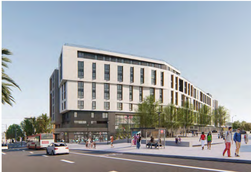
Exterior Façade adjacent to BART Plaza
