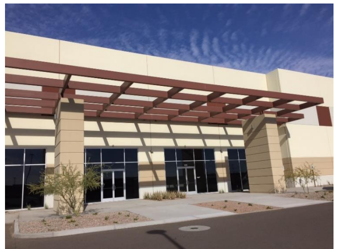
LAI Southwest expansion in Tempe, AZ
