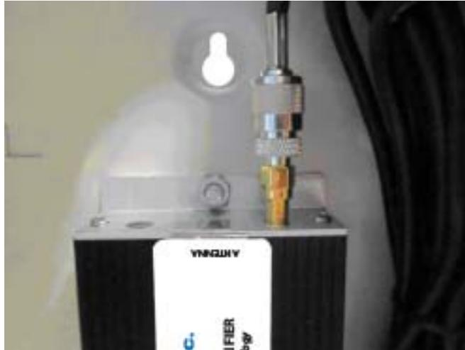
5. Mount the Outdoor Signal Antenna vertically on the enclosure metal surface. Antenna must be located in the same room as the amplifier and the cellular communicator.
