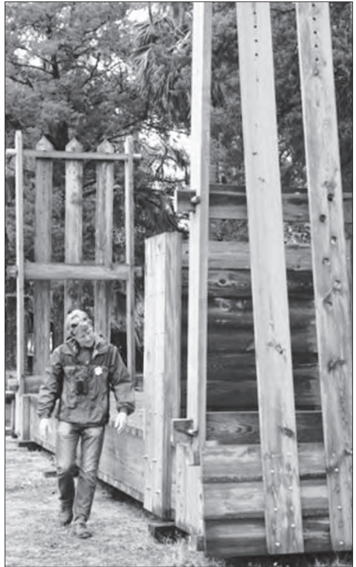
Dr. Patrick McMillan examines a newly constructed rice trunk at Nemours Plantation.
