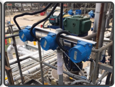
Multiple smartPIMS® Modbus DSIs networked for monitoring dozens of TMLs.
