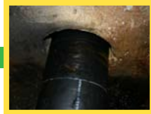
Short lengths of pipe, lowered down the manhole one at a time.
