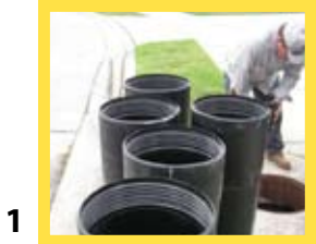
Thread-Liner is manufactured in short lengths for easier installation.
