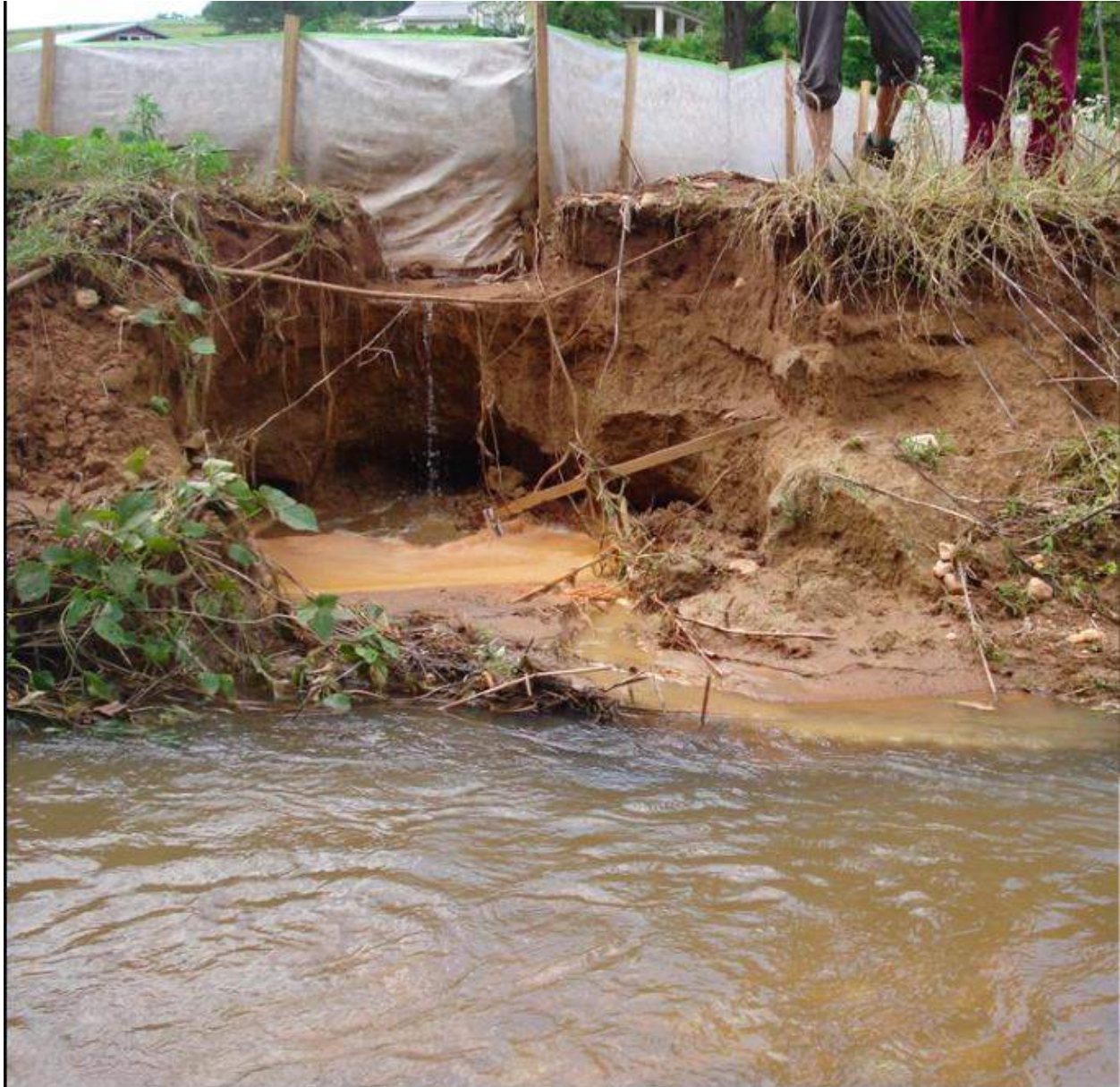
Fig. 3 – Bernard property, May 20, 2018 (looking across Teals Creek to the northeast; tributary enters Teals downstream and to the right from this spot.) This is the same location as shown in Fig. 3. New measures have been installed but very heavy sediment discharges continued in June.
