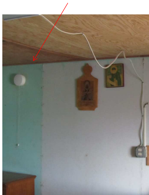
New ventilation intake
