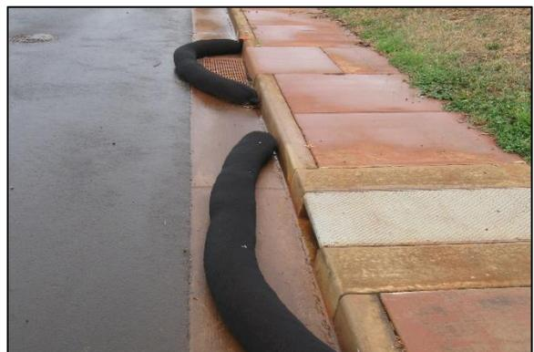
**Myth No. 4: Fibre rolls/logs should always be installed on top of an Erosion Control Blanket.**
