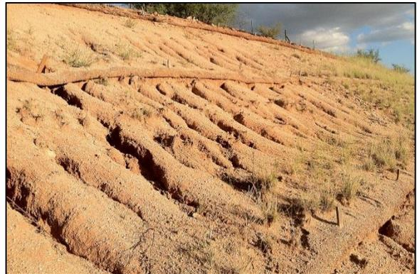
**Myth No. 2: Spacing of hillside fibre roll/log barriers is not important.**
