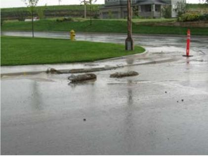
Today, a multi-million dollar industry provides a variety of products created to meet EPA's mandate of installing construction site BMPs to "minimize pollutants" in the discharge of runoff waters. A common use of barriers is their installation in front of curb inlets---which can divert runoff and cause *downstream flooding*.
