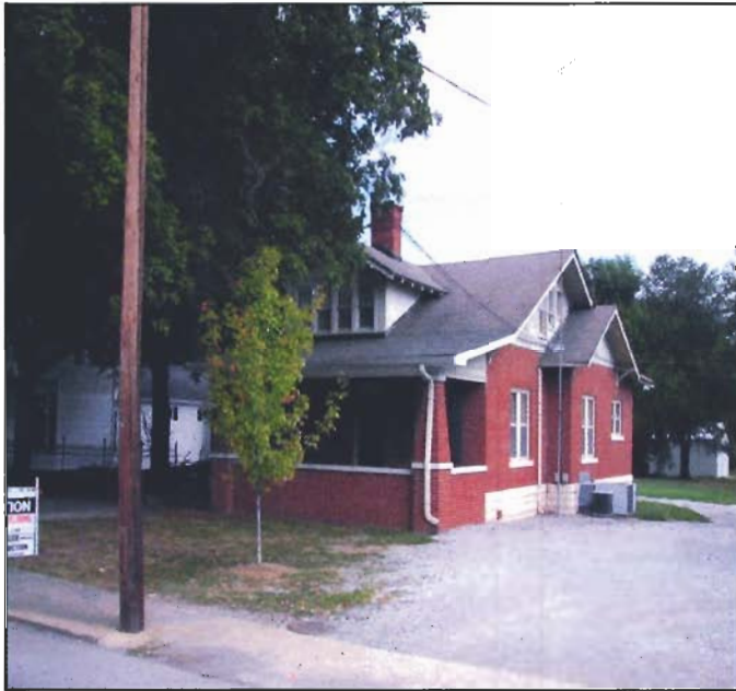
Front View of 1-1/2 Story Office Building
