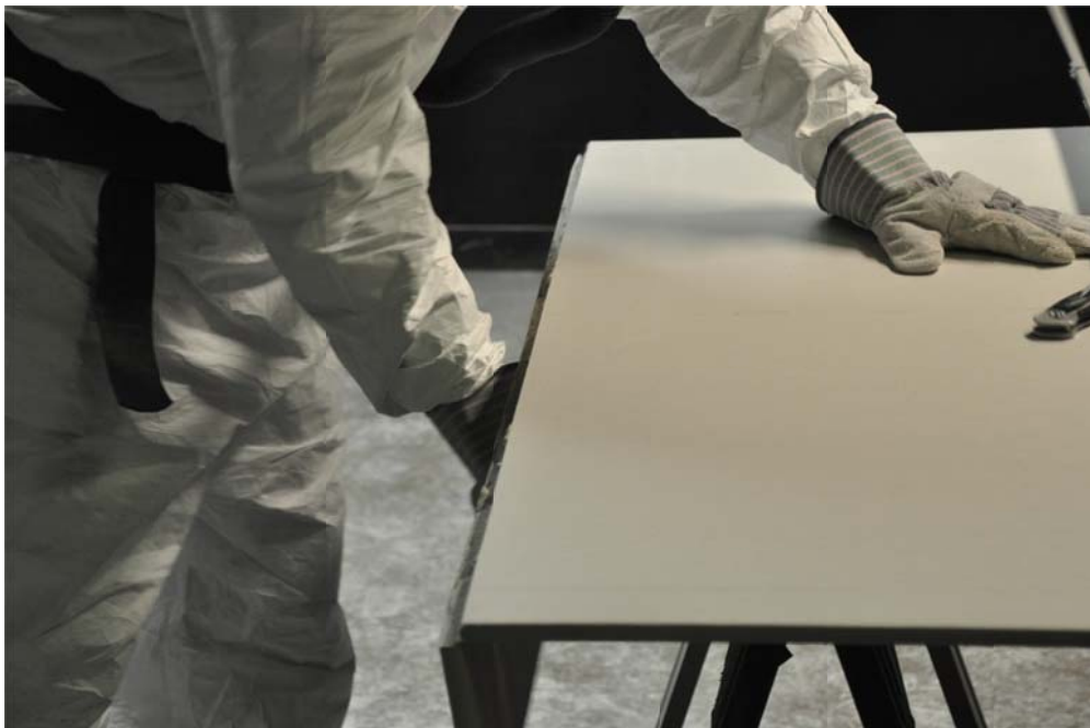
Figure 5. Snapping a 5/8" Type X drywall board using downward hand force.
