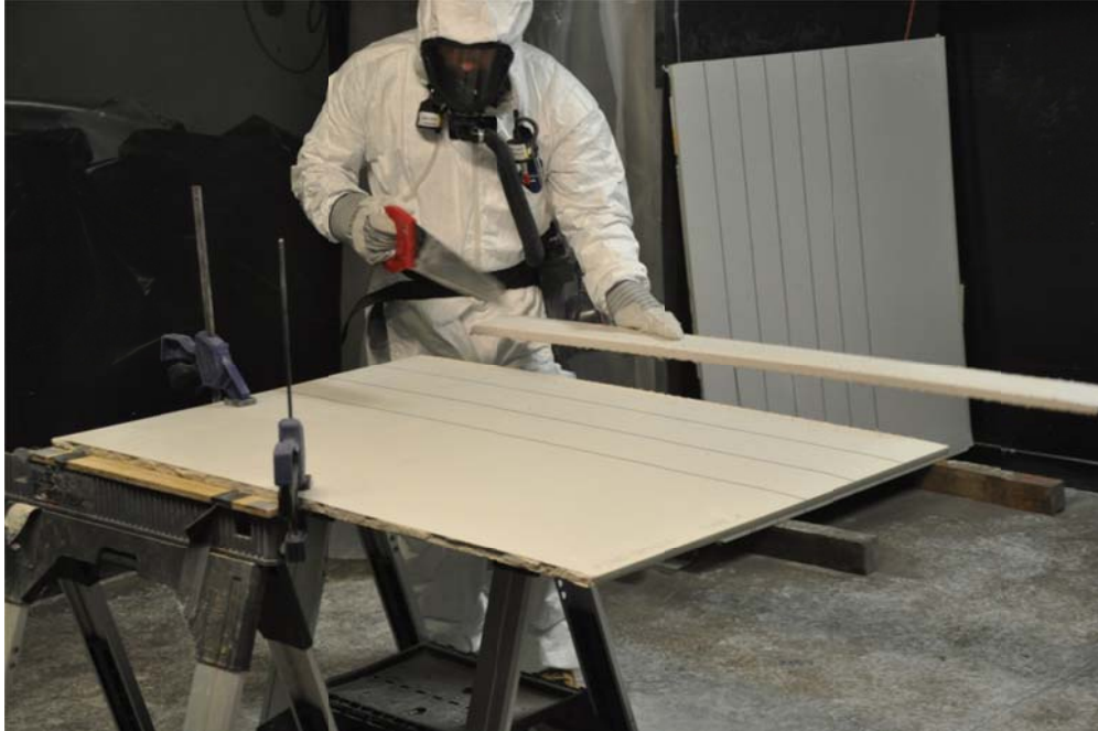
Figure 8. Cutting a 5/8" Type X drywall board section with the hand saw.
