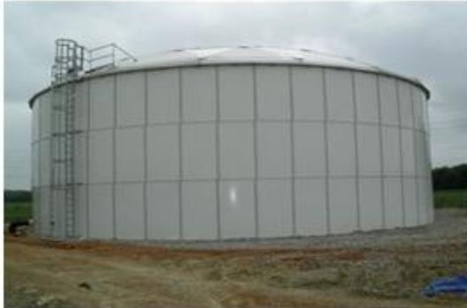
**Figure 4: Fire protection water storage tank.**
