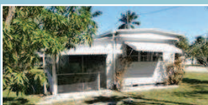
MAKE OFFER Intersecting canal to Matlacha Pass with mobile & guest house. Needs TLC. $189,900
