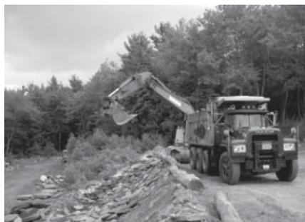
be weighed. Wall stone is sold by weight (a typical dump truck full is 20 tons).
