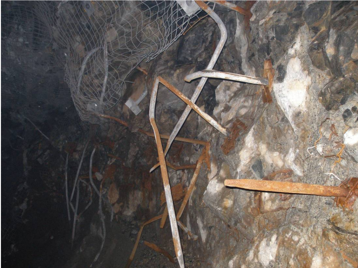
Figure 10: Condition of the up dip exposure at 465 before shotcreting.
