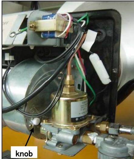
1. Unfasten a knob and expand combustion air inlet opening.
