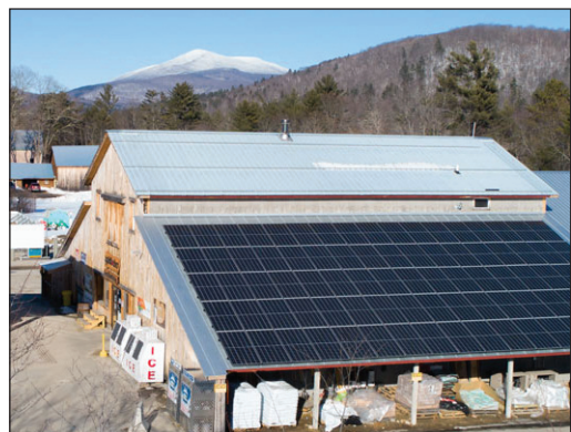
NH Solar Shares' second community solar PV array is located on the roof of Appleknockers General Store in Warren.
