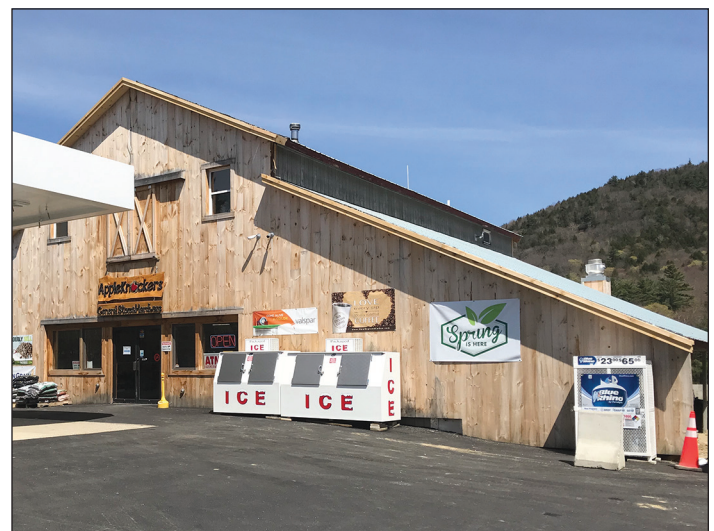
NH Solar Shares' second community solar PV array will be located on the roof of Appleknockers General Store in Warren.
