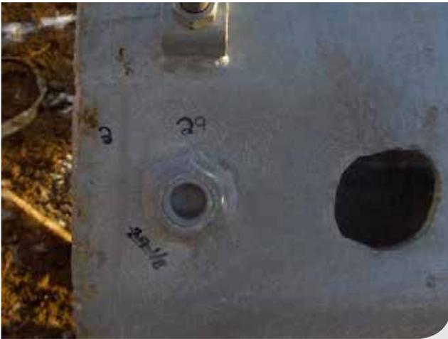
Slip Joint Jacking Bolt and Inspection Hole
