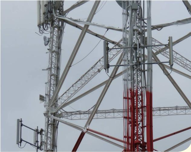
*Large SSV with antenna or lighting install at mid-point.*
