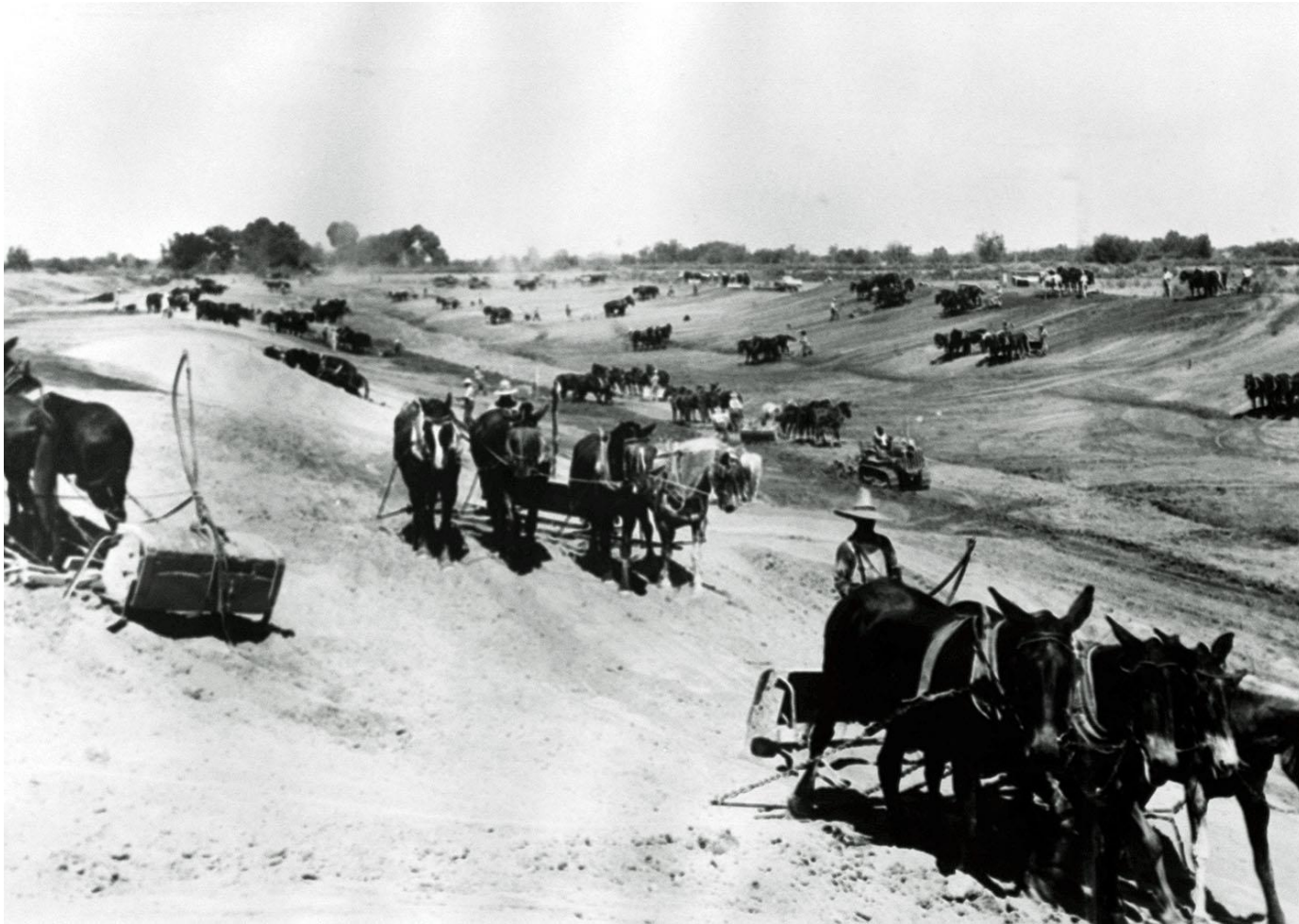
Excavation of the All American Canal by government force, 11 July 1935
