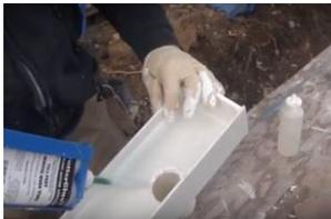
Outlet should be a tight fit to gutter. If it is loose or will not sit straight use 2P10 Superglue to hold it in place while applying final bonding agent.
