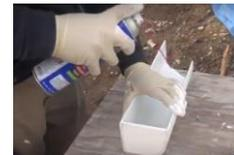
Stick Endcap in place so that it is flush with edge of gutter
