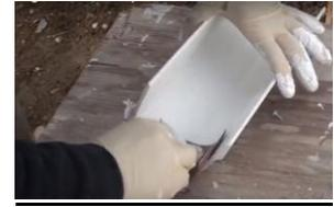
Sand any bonding surfaces where the endcap is to be installed (including on the gutter).
