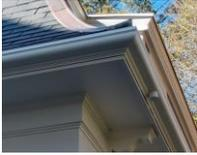
(Leave enough space for downspout to fit between outlet and fascia)
