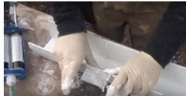
Wet out Fiberglass Cloth with GutterGlue and lay into Miter/Seam.
