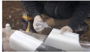
Wipe with acetone and use 2P10 superglue (recommended) to temporarily hold seam together
