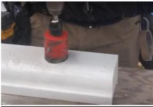
Drill through gutter with a 2-3/8" hole saw
