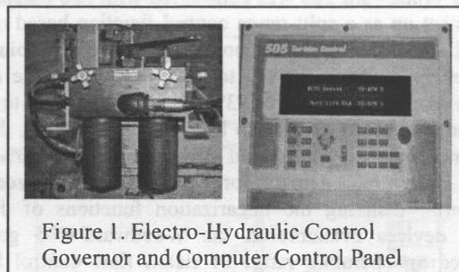
Figure 1. Electro-Hydraulic Control Governor and Computer Control Panel
