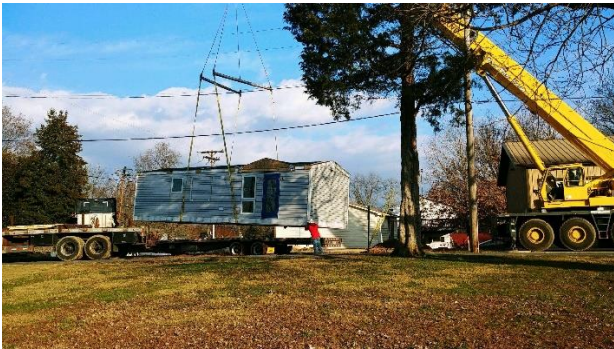
Photos of the new Post Office being installed.
