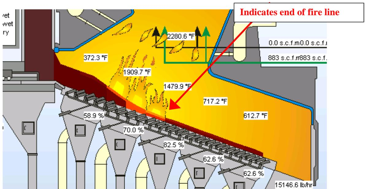
Figure 2: Furnace profile showing fire line
