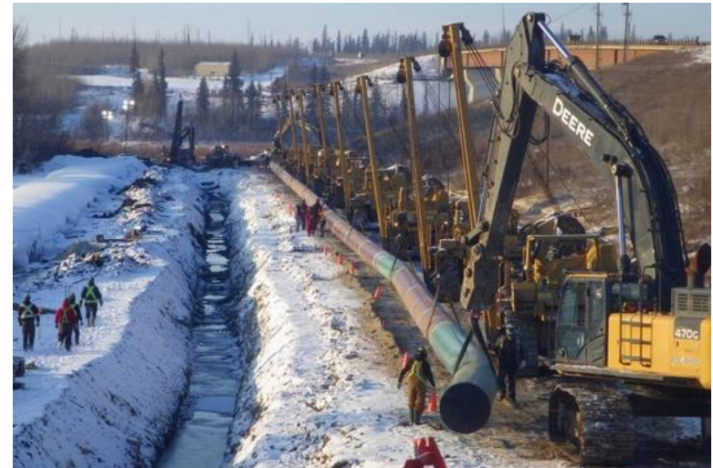
Lowering in 36" pipeline at Beaver Pond 2016
