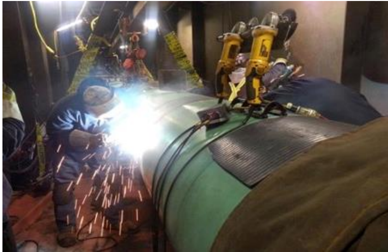
Welding in tight area under bridge 2016
