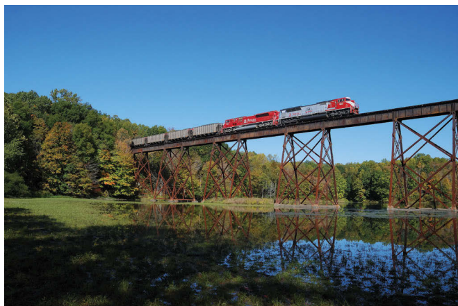
Shuffle Creek Trestle is 982 feet long and stands 80 feet over the swampy shallows of Lake Lemon.
