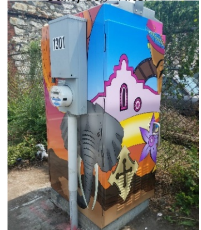
Utility Box - After
