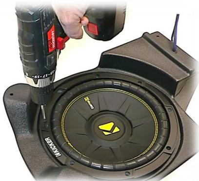
Use (8) provided black subwoofer screws to affix sub to pod, **starting** with a drill w/ phillips bit....
