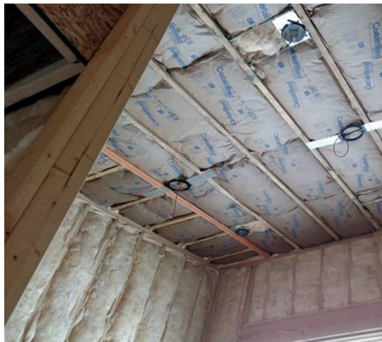
Custom-home builders and contractors rely on Buday's for their expertise, quality, and reliability. This photo shows how our professional installers install wireless access points prior to the installation of drywall.
