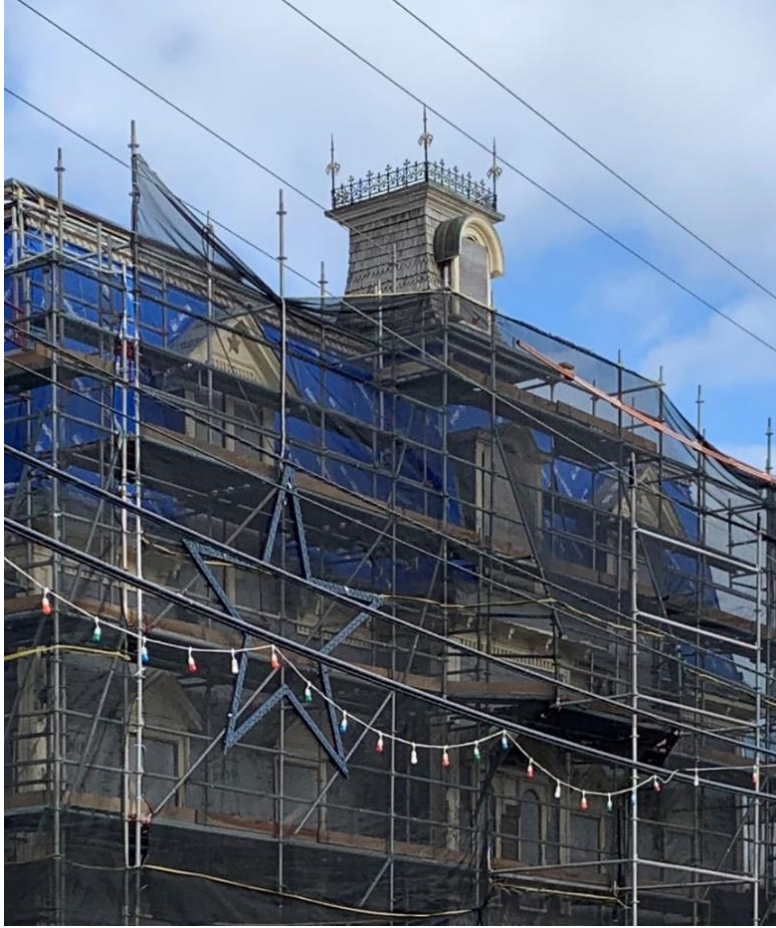
Building Stabilization Efforts Continue
