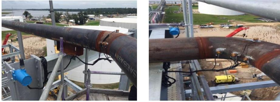
**Figure 10: Crude unit overhead line corrosion monitoring at 300-degrees F using dual-element transducers and cellular back-haul.**
