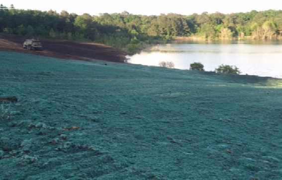
ProGanics and Flexterra applied to soil in April
