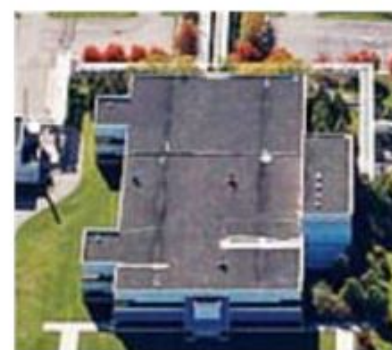
640 Building Former Data Center
