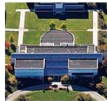
600 Building Hospitality Building
