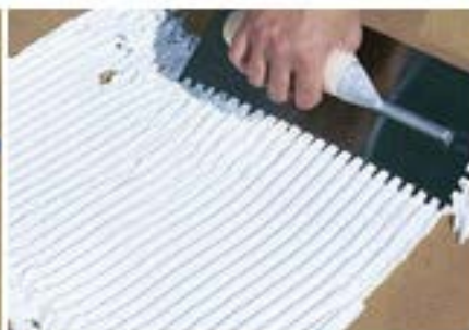
Apply thinset with a trowel.
