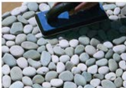
Lightly tap down the tile without pushing the pebbles into the thinset.
