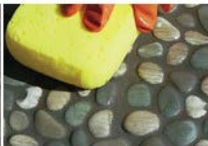
Repeat sponging off the grout until the desired look is reached. Look for narrow grout lines between the pebbles. Once the grout has completely dried seal the tiles a final time.
