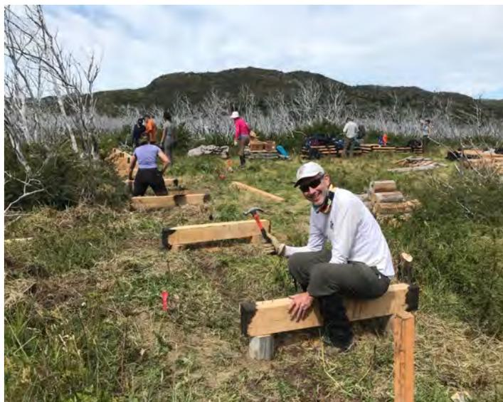
Two stringers were placed per each seven-foot section and secured with metal brackets. Once the stringers were in position, the decking was secured with self-tapping screws. The final touch was trimming the boards to provide an aesthetically pleasing boardwalk.
