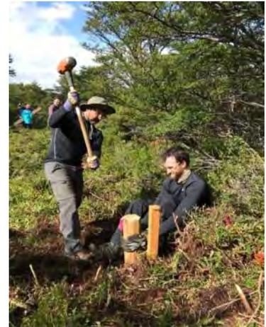
Once the posts were secured and leveled, a beam was attached to the post and leveled to hold the stringers.
