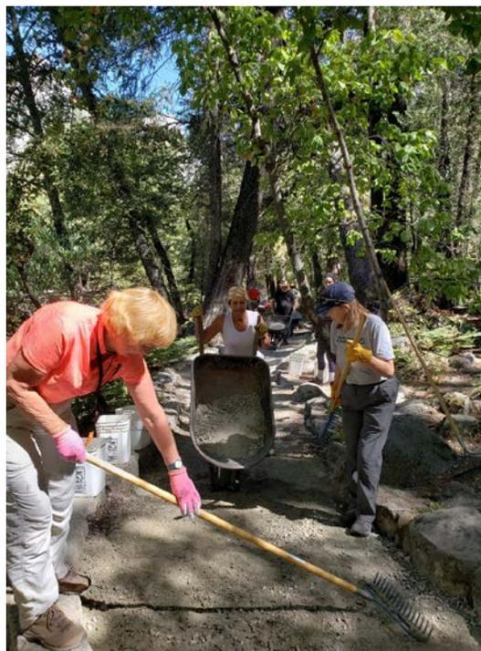
Using wheelbarrows, teams of volunteers moved 8 to 10 tons of specially constructed road-base from a stockpile near the nature center to the work site. Once deposited, volunteers raked the material into place, building up the trail surface 3-inches at a time. Others sprinkled the newly placed road-base with water from the Merced River so that the material could be compacted with a vibratory plate compactor (also wheeled to the
