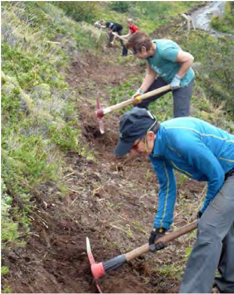
Building 800 feet of new trail tread leading to the suspension bridge
