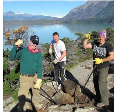
*Trail Resurfacing:* In some areas the trail tread was made up of loose boulders, making it awkward and unsafe for hikers. Approximately 80-feet of such trail were resurfaced. Dirt was filled in over small to medium-size boulders, resulting in a smooth, safe hiking surface. Approximately 20-feet of slough removal was completed to raise trail tread for water shedding.
