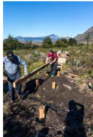
Initially, making the vertical posts was very time consuming, as it was a one-person job, cutting cypress logs into 3-4 foot pieces using a brushing saw, and then sharpening one end with an axe. On the third afternoon, CONAF delivered a chain saw for our use, and this greatly simplified and sped up the process. The stringers and decking required only occasional cutting to length.
