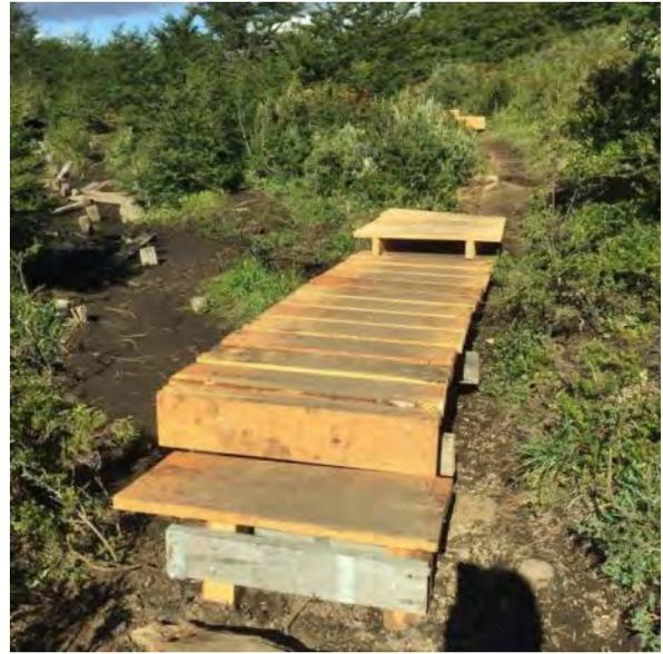
In addition, 90 feet of existing boardwalk was refurbished. Refurbishing the existing boardwalk consisted of rebuilding the decking utilizing used material scavenged from piles of discarded materials that were nearby. Finding good material took time, but in the end, a good boardwalk was assembled.
