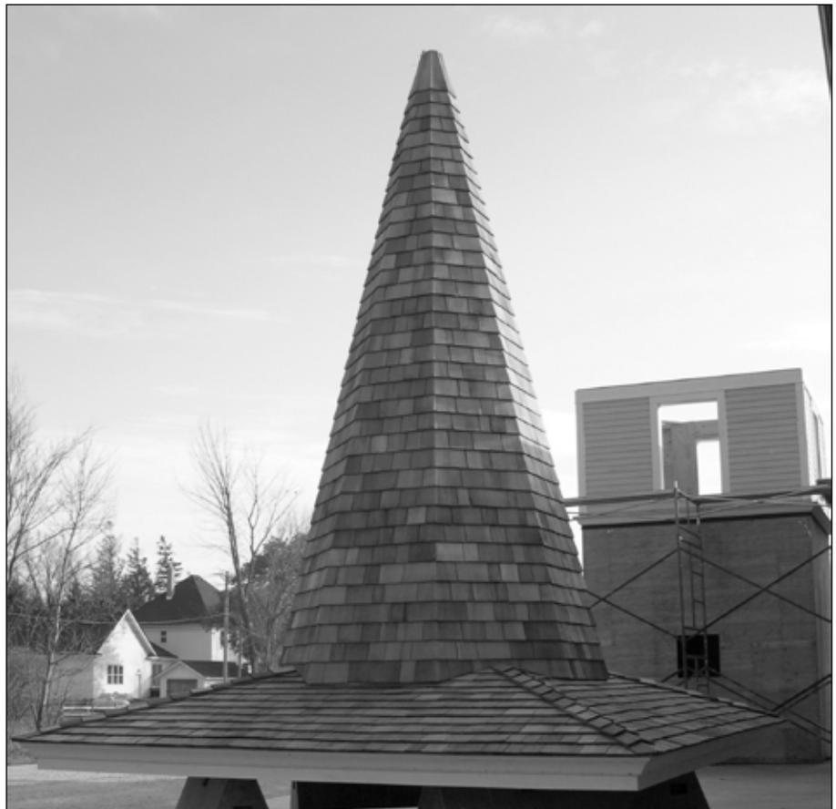
November 16<sup>th</sup>: With proper footings, new columns, replaced and reinforced beams, the new steeple was craned into place with only 1½ inches clearance between the church roof and edges of the steeple. With little wind, the start to finish of the crane's time installing the steeple was two and a half hours.
